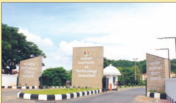
Newly constructed main gate of IIT Guwahati
